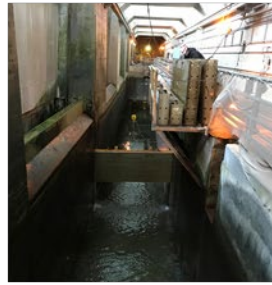
c. Dewatering bulkheads
